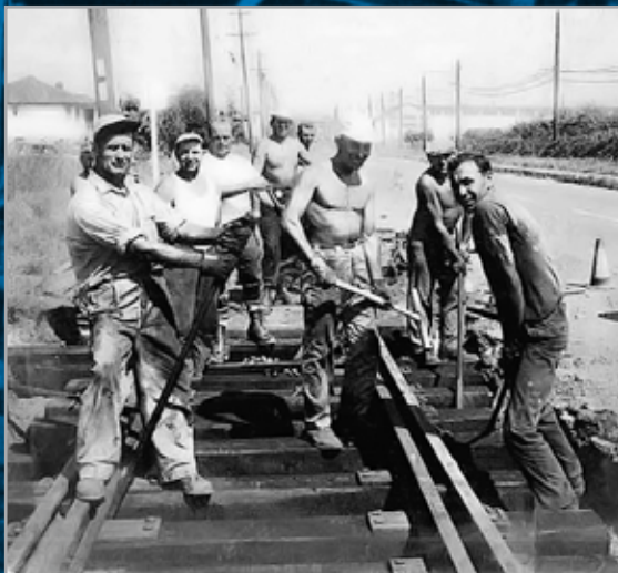
A crew constructs track in the 1960s in Langley, British Columbia, to connect the newly constructed Delta Port to Canadian Pacific Railway main line track.
