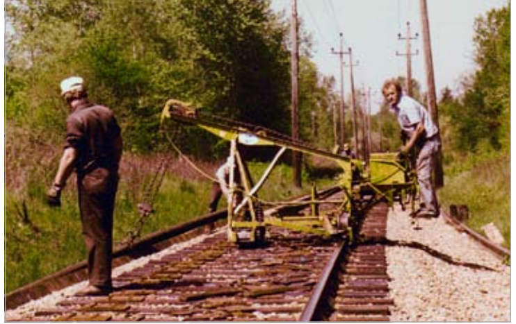
A crew changes rail for BC Hydro in Langley, British Columbia, in 1983.
