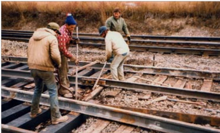
A crew rehabilitates track in the 1980s.
